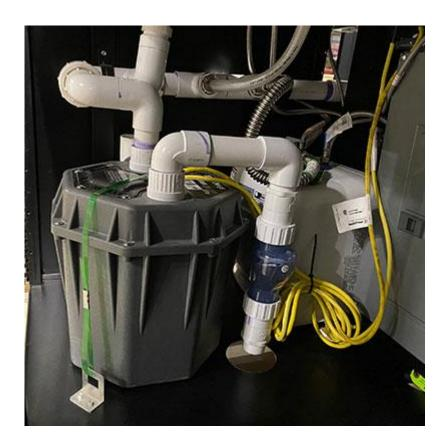
Sanitary for the Enhanced Pop-Up Store is provided using Drain Pumps located in the Utility Compartment of each Rear Cart. These Drain Pumps are  $\frac{1}{2}$ -HP and has great head height (up to approximately 35 feet) and supports high temperatures (up to 180F).
