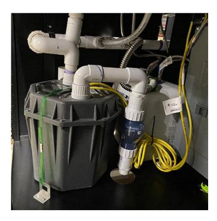
Sanitary for the Starbucks Standard Plus Store is provided using a Drain Pump located in the Utility Compartment of the Main Rear Cart. This Drain Pump is 1/2HP and has great head height (up to approximately 35 feet) and supports high temperatures (up to 180F).
